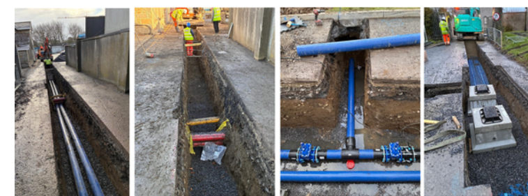
Water and Fire Main Project
